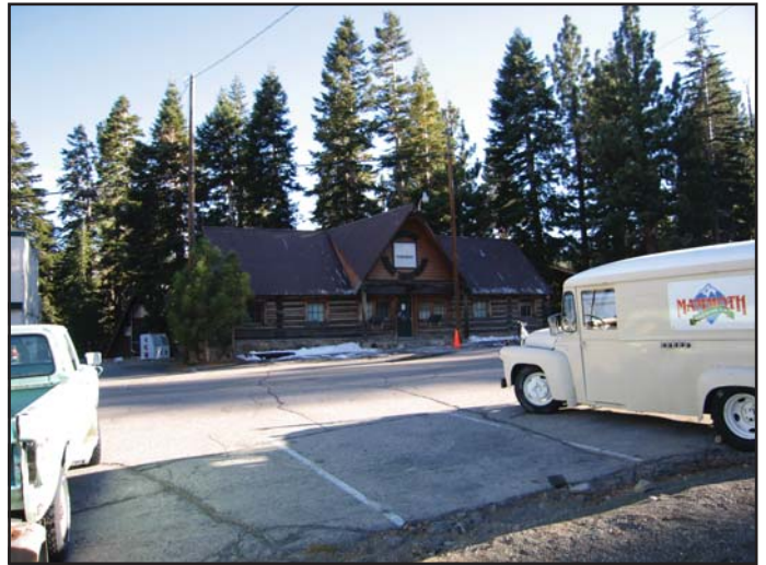
View 5: Looking southwest towards Site 2 from Lake Mary Road.
